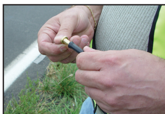
Put End Plug in the end of tube.
