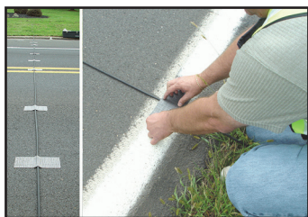
Tape the tube down with mastic tape at multiple spots.
