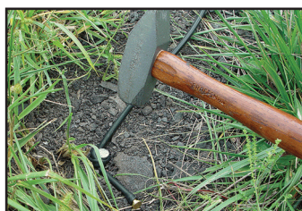
Secure the tube to the far side of the road.
